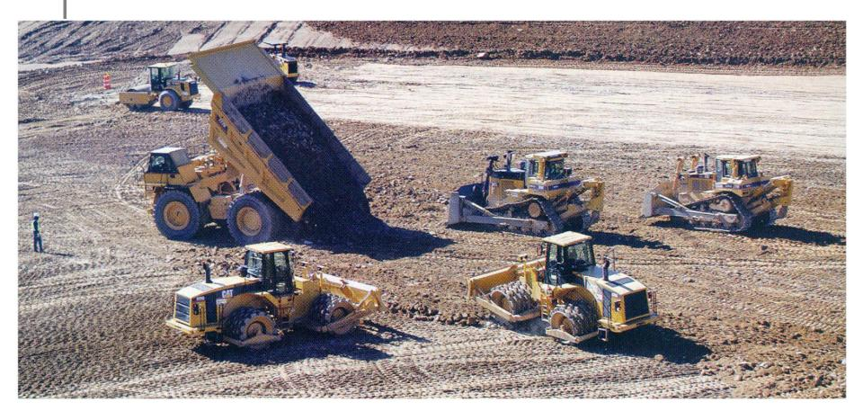
Motor-scarifier cuts and lays fills in 8 to 24 inch lifts for compaction
