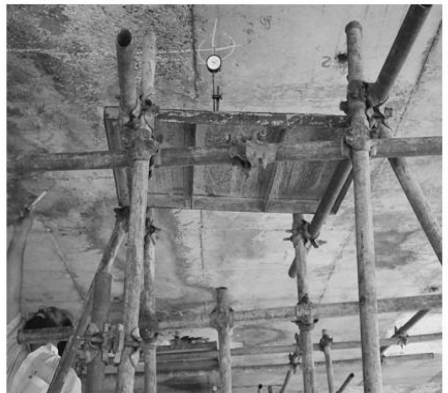
Fig. Deflection Gauge Installed at the Center of Panel
