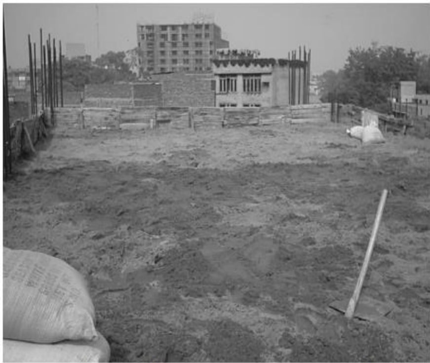
Fig. Load Application with Loose Sand within Wooden Shuttering.
