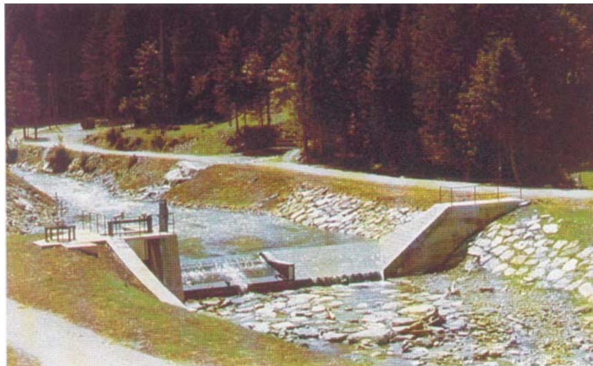
Fig. 2.21: Tyrolean weir in Austria [22]
