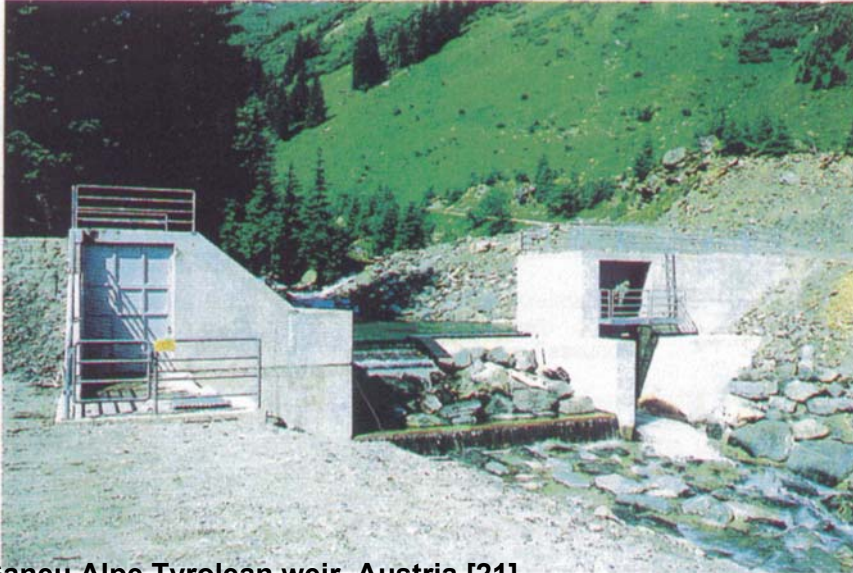
Fig. 2.20: Ganeu Alpe Tyrolean weir, Austria [21]
