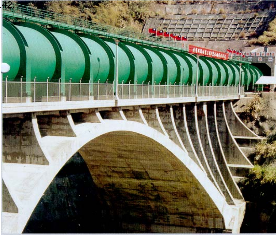
Fig. 2.42: Location of a pipe bridge over rugged terrain [1]
