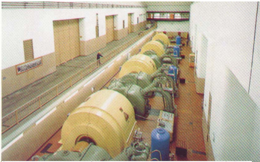
Fig. 2.69: Example of Francis turbine with horizontal shaft [27]
